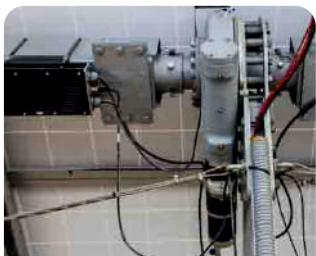
Improper Cabling
